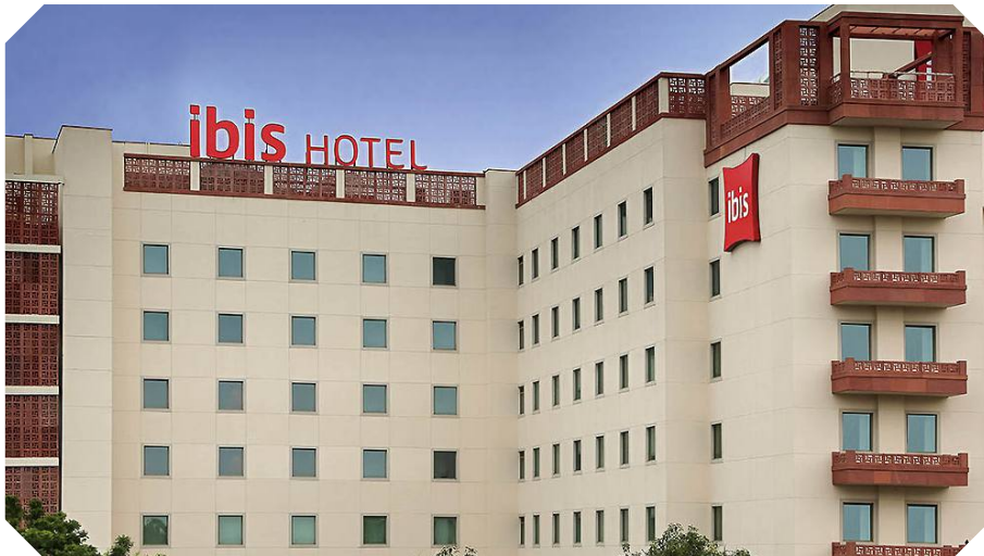
Hotel IBIS - Jaipur HVAC | Value - 2.19 Cr. Approx
