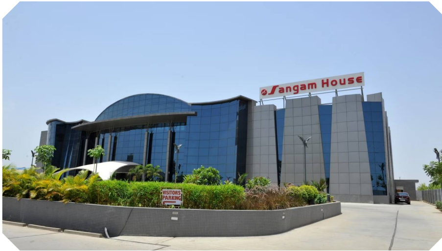
Sangam India Ltd - Bhilwara HVAC, Fire Fighting | Value - 3.00 Cr. Approx
