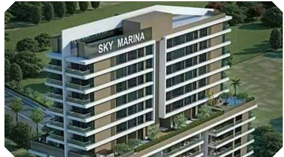
SKY Marina - Udaipur HVAC, Fire Fighting | Value - 2.50 Cr. Approx
