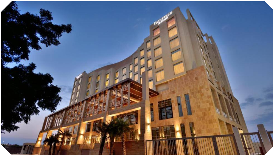
Fairfield Inn & Suites By Marriott - Jodhpur HVAC | Value - 5.82 Cr. Approx
