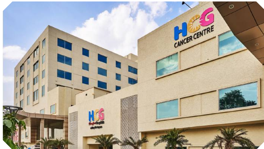
HCG Mangalam Hospital - Jaipur HVAC, Fire Fighting | Value - 11.00 Cr. Approx
