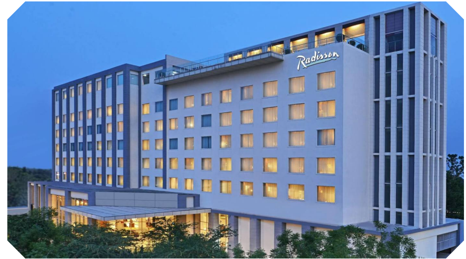
Hotel Radisson - Dhanbad (Jharkhand) HVAC, Fire Fighting | Value - 5.00 Cr. Approx
