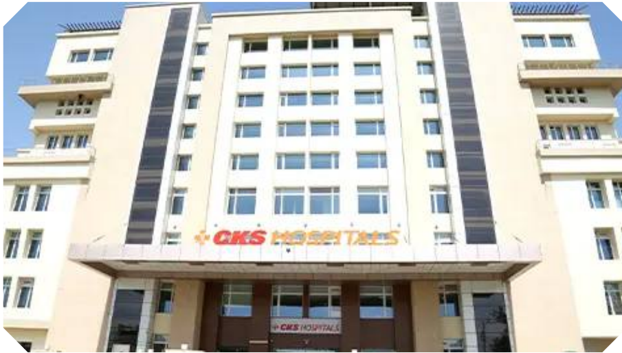
CKS Hospital - Jaipur HVAC | Value - 4.08 Cr. Approx
