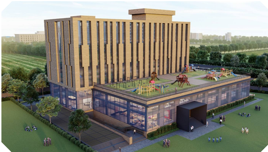
Neerja Modi School - Jaipur HVAC | Value - 1.50 Cr. Approx
