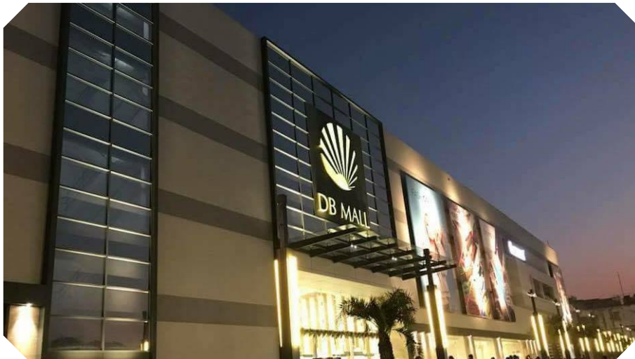
DB Mall - Gwalior HVAC | Value - 3.20 Cr. Approx
