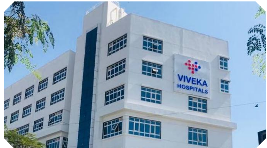
Viveka Hospital - Nagpur HVAC | Value - 5.95 Cr. Approx
