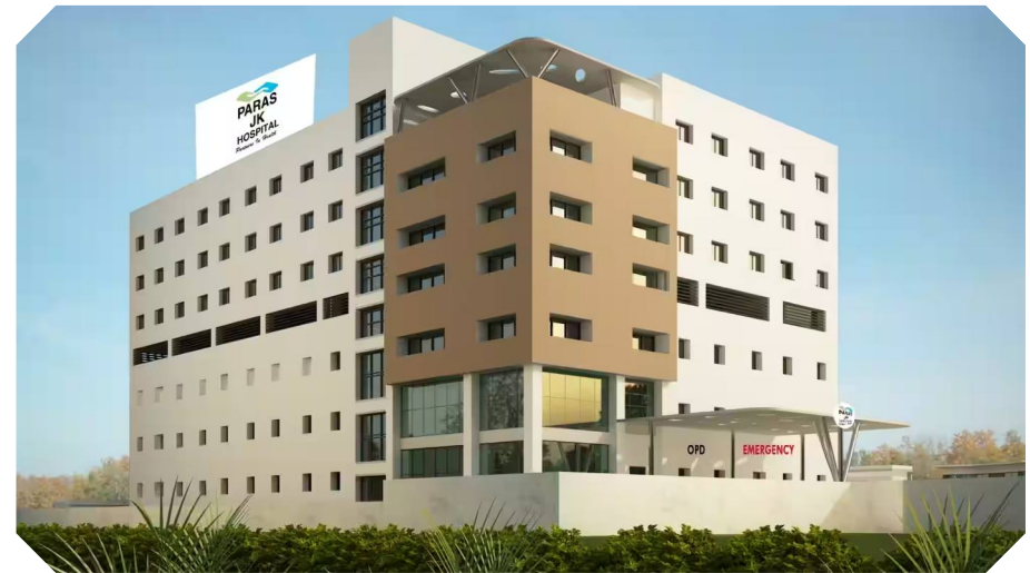
Paras JK Hospital - Udaipur HVAC, Fire Fighting | Value - 6.22 Cr. Approx
