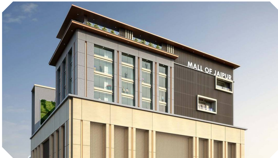
Mall of Jaipur - Jaipur HVAC, Fire Fighting, BMS | Value - 14.00 Cr. Approx
