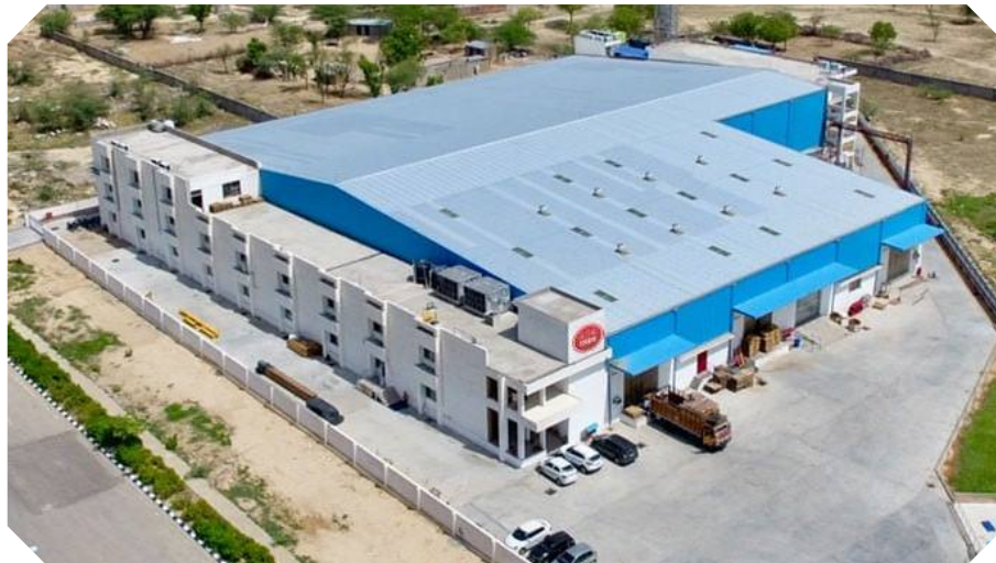
Alisha Torrent Closures India Pvt. Ltd. - Jaipur HVAC, Fire Fighting | Value - 4.05 Cr. Approx
