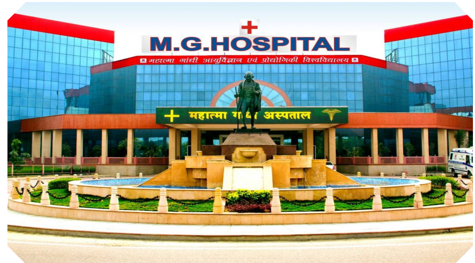
Mahatma Gandhi Hospital - Jaipur HVAC, Fire Fighting | Value - 20.50 Cr. Approx
