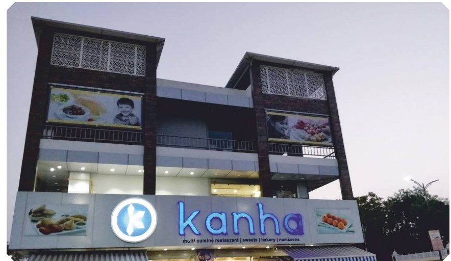
Kanha Industries - Jaipur HVAC, Process Cooling | Value - 3.25 Cr. Approx
