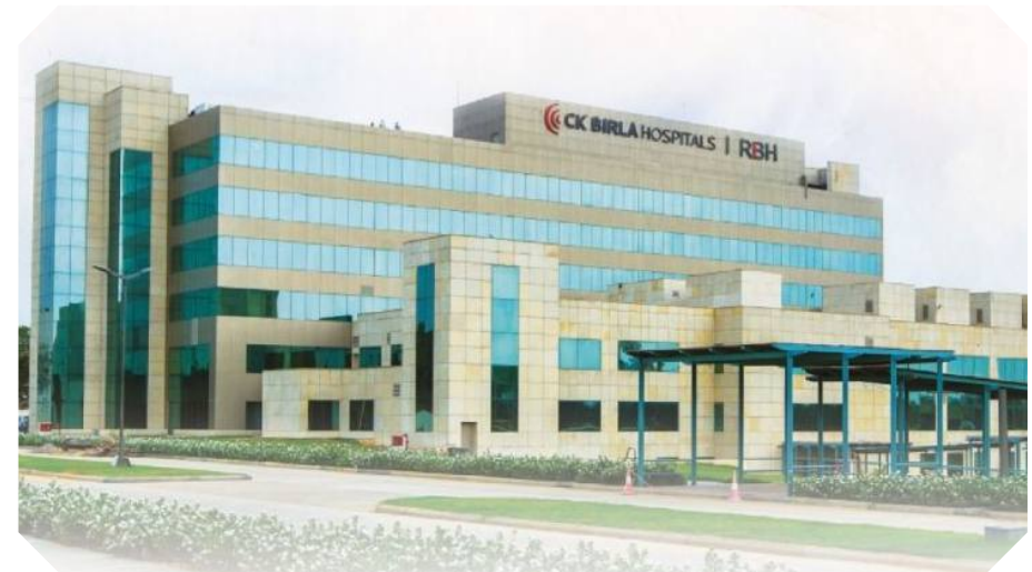
C.K. Birla Hospital - Jaipur HVAC, Fire Fighting | Value - 15.65 Cr. Approx
