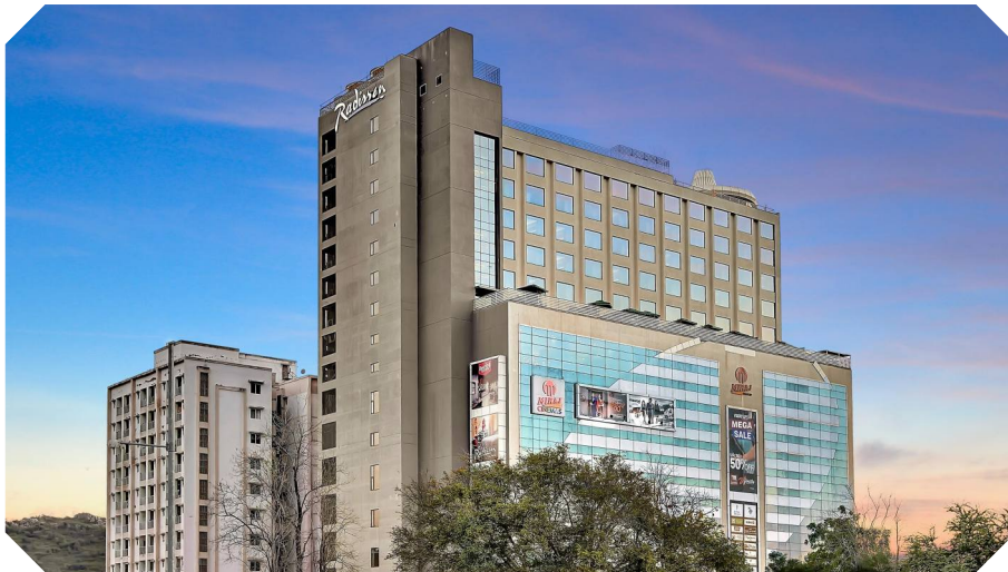
Radisson Hotel & Miraj Mall - Nathdwara HVAC | Value - 6.50 Cr. Approx
