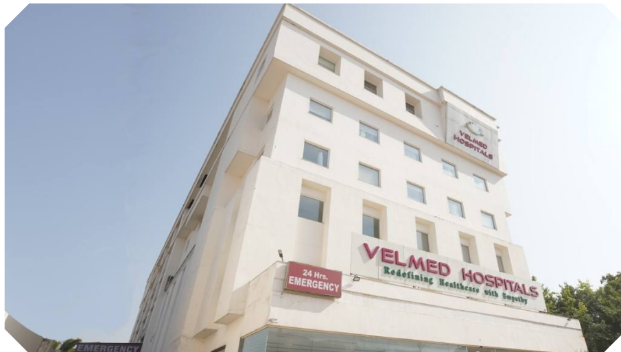
Velmed Hospital (Bharat Heart Institute) - Dehradun HVAC | Value - 6.05 Cr. Approx
