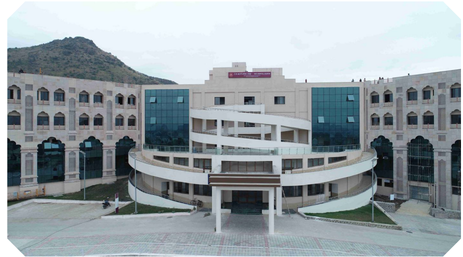
ESIC Hospital - Udaipur HVAC, Fire Fighting | Value - 3.02 Cr. Approx
