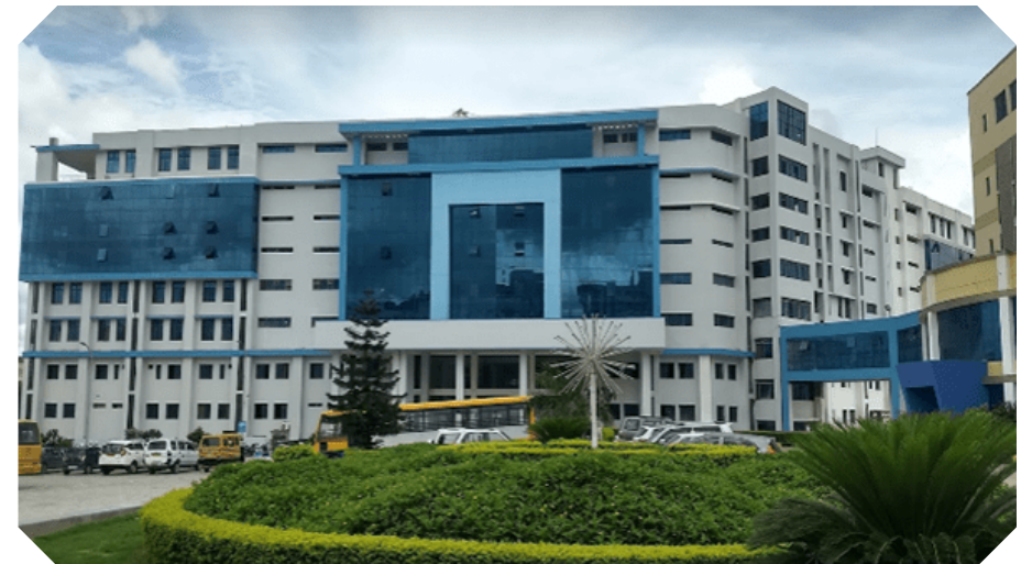
GBH American Hospital & Medical College - Udaipur HVAC, Fire Fighting | Value - 10.00 Cr. Approx
