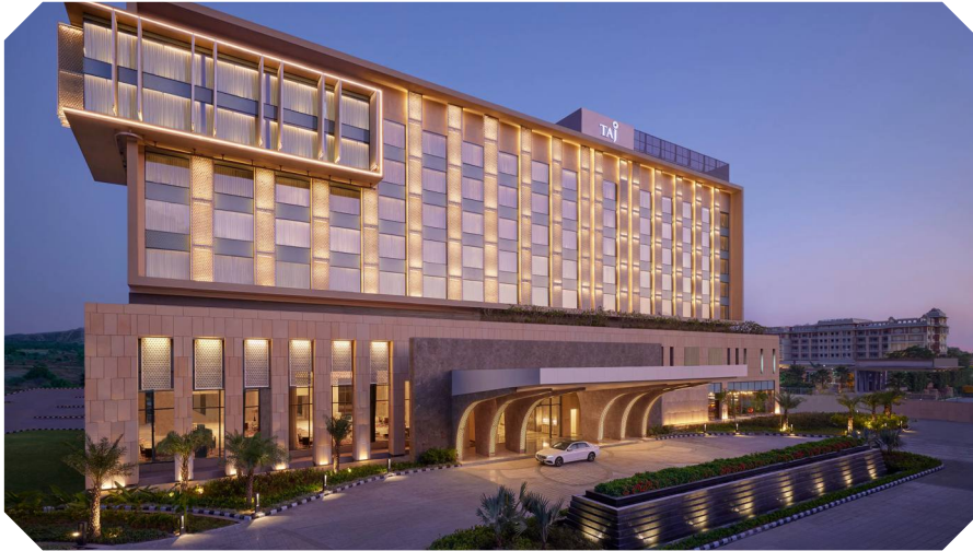
The Taj - Amer - Jaipur HVAC | Value - 10.00 Cr. Approx
