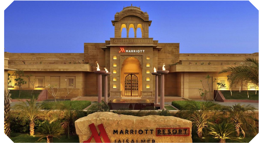
Marriott Resort & Spa - Jaisalmer HVAC | Value - 6.02 Cr. Approx
