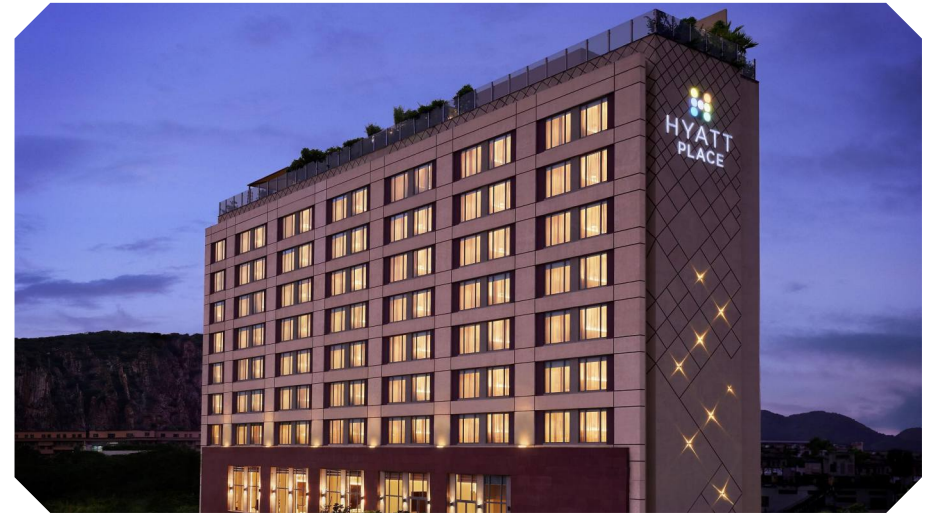
Hyatt Place - Jaipur HVAC, Fire Fighting, Electrical, Plumbing Value - 10.25 Cr. Approx
