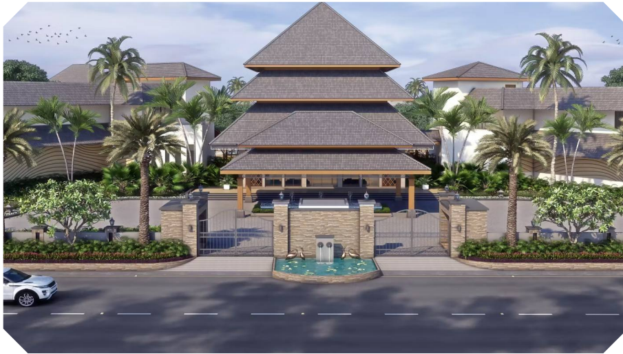
Westin Resort & Spa - Jaipur HVAC, Fire Fighting | Value - 5.40 Cr. Approx
