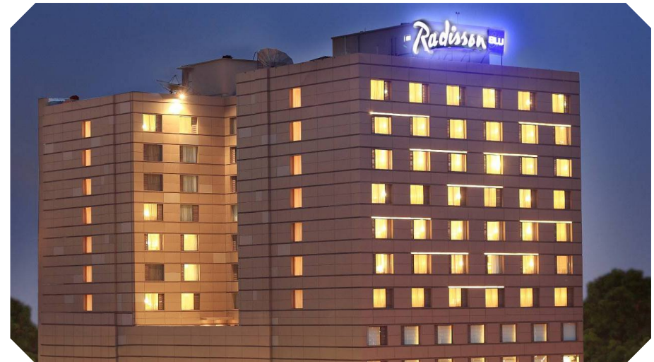
Radisson Blu - Dehradun HVAC, Fire Fighting | Value - 6.00 Cr. Approx
