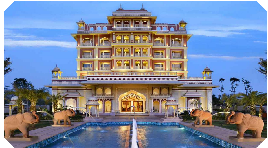
Hotel Indana Palace - Jaipur HVAC | Value - 3.56 Cr. Approx
